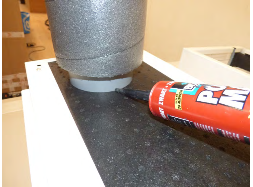
Figure 12 Slide the insulating cover over the duct pipe – use Polymax to make an air tight connection
