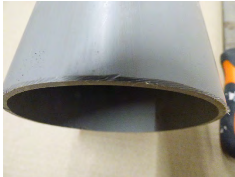
Figure 7 Deburr and chamfer the duct pipes making insertion into the white ring possible
