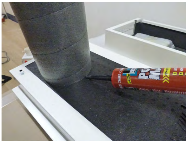
Figure 14 Internal wall sealing
