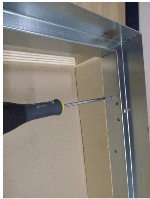
Figure 5 Fasten the bottom U shape with the screws provided
