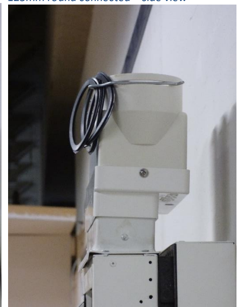
Figure 36 Adapt and Radial 3 X 75 connection piece direct to adapter flange
