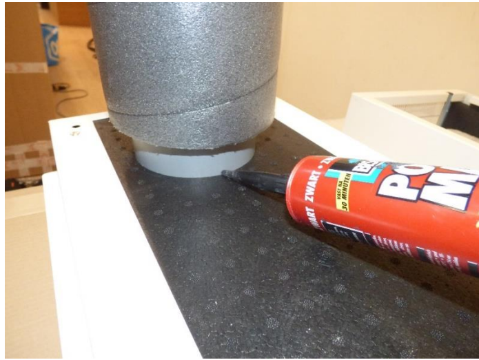
Figure 22 Slide the insulating cover over the duct pipe – use Polymax to make an air tight connection
