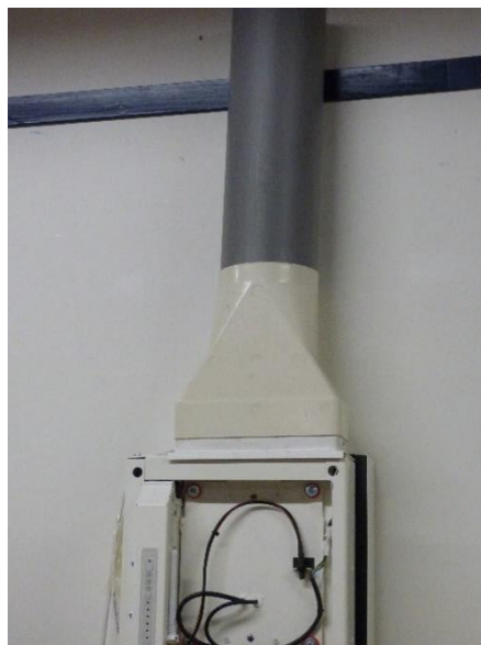
Figure 34 Square to round adapter with 125mm round connected
