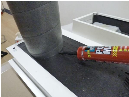
Figure 24 Internal wall sealing
