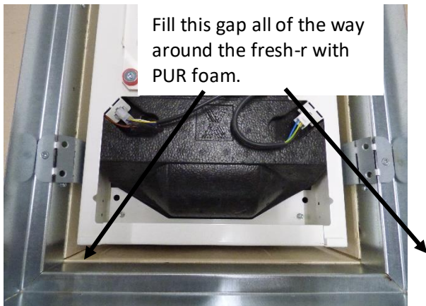
Figure 41 Insulate between fresh-r and installation frame
