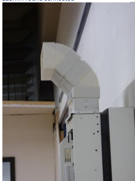
Figure 37 90 degree bend using 2 X 45
