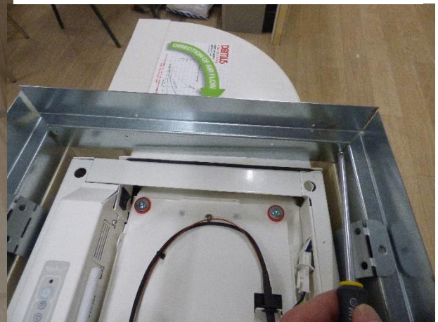
Figure 29 Fresh-r everywhere with duct connection and closed top
