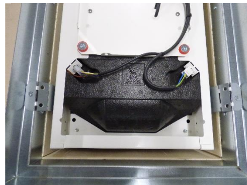
Figure 26 Lower end of fresh-r properly secured
