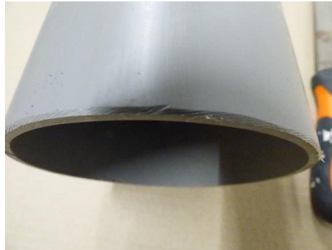
Figure 17 Deburr and chamfer the duct pipes making insertion into the white ring possible
