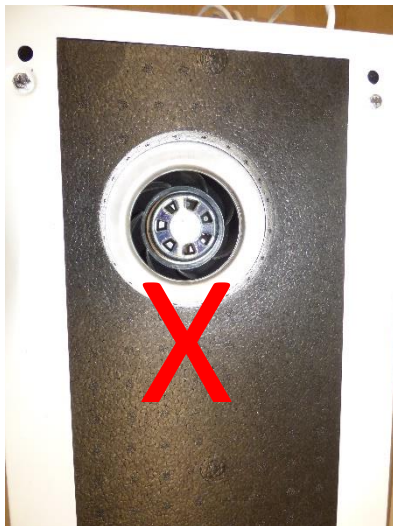
Figure 19 DO NOT USE PCV GLUE Top of Fresh-r unit
