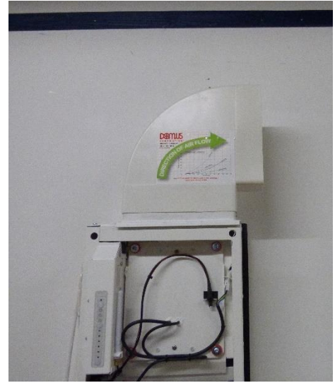
Figure 31 Low loss bend fitted directly onto adapter
