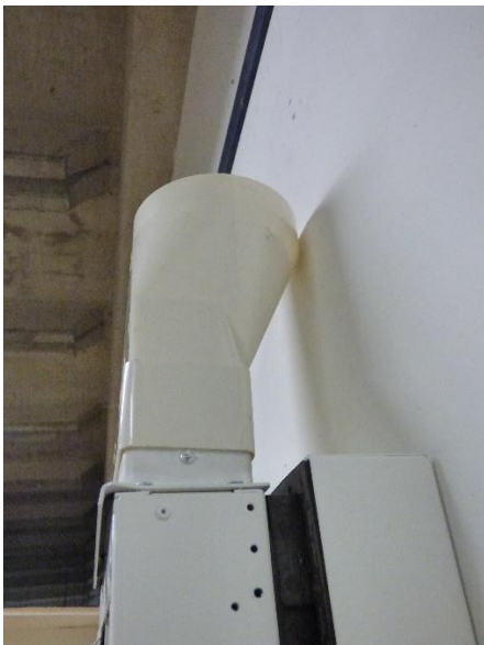
Figure 35 Square to round (125mm) fitted directly to adapter
